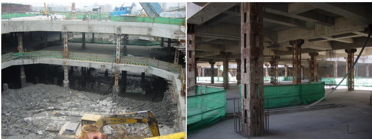
Fig.7.7 Inside the excavation and details of retaining structure (Xu 2007)
